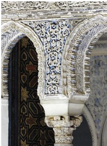
Construction materials: wood (doors), plaster (arches), marble (columns and capitals)
