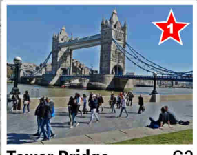
1 Tower Bridge G3
