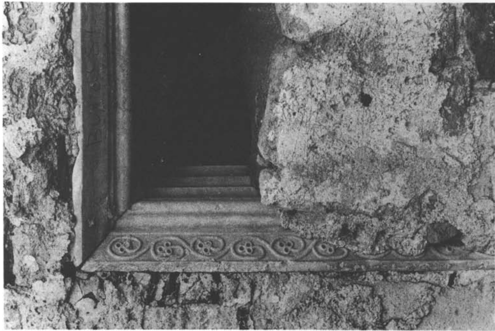
29 Enez. Inner narthex, south portal. Detail of lintel
